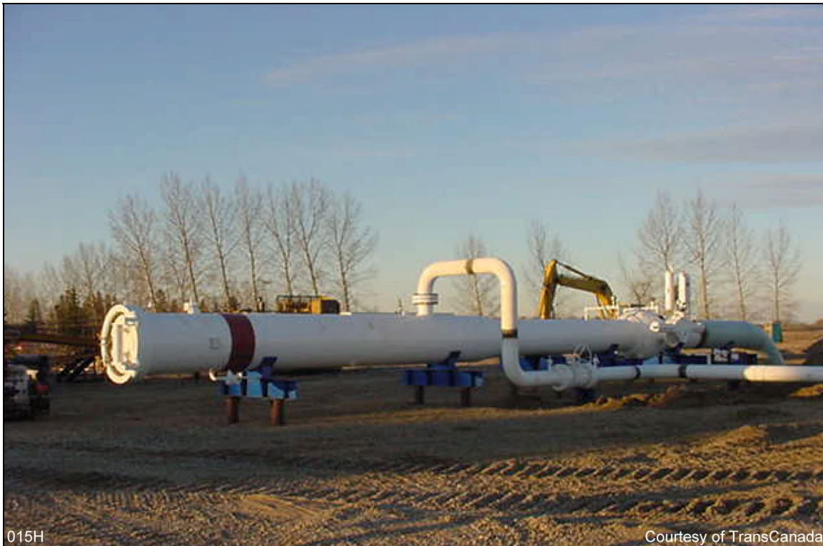
Figure 3-16: Example of a Pig Launcher or Receiver
