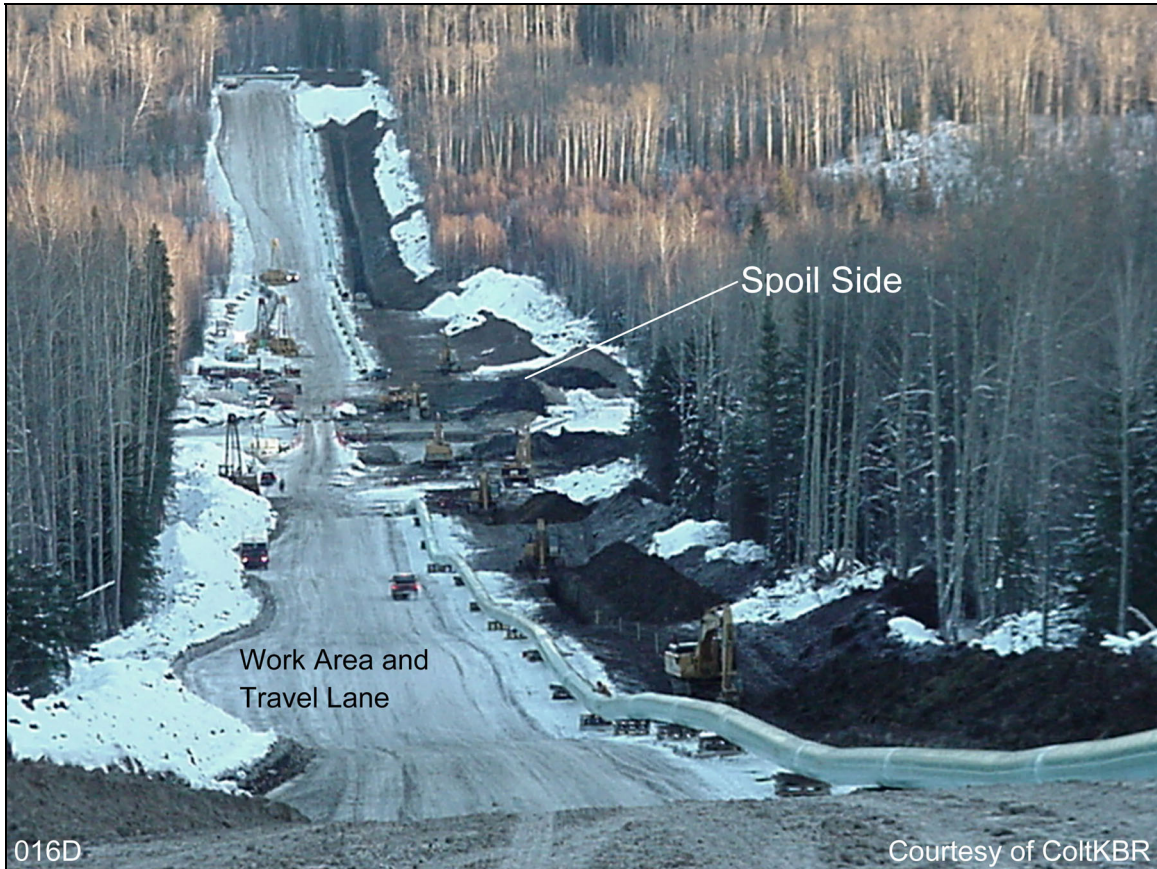
Figure 3-5: Example of Right-of-Way with Travel Lane
