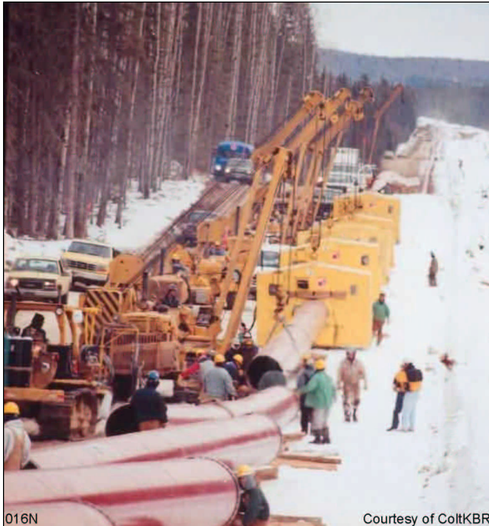
Figure 3-21: Example of a Right-of-Way During Construction
