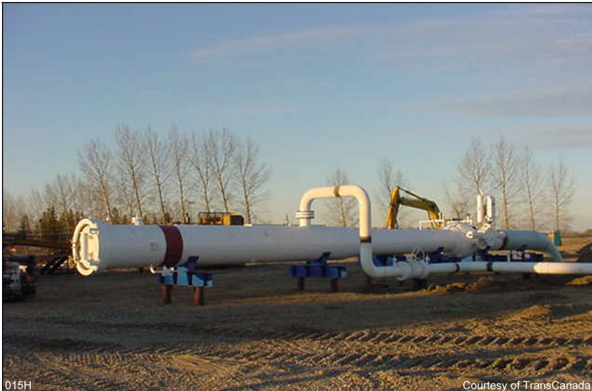
Figure 3-16: Example of a Pig Launcher or Receiver
