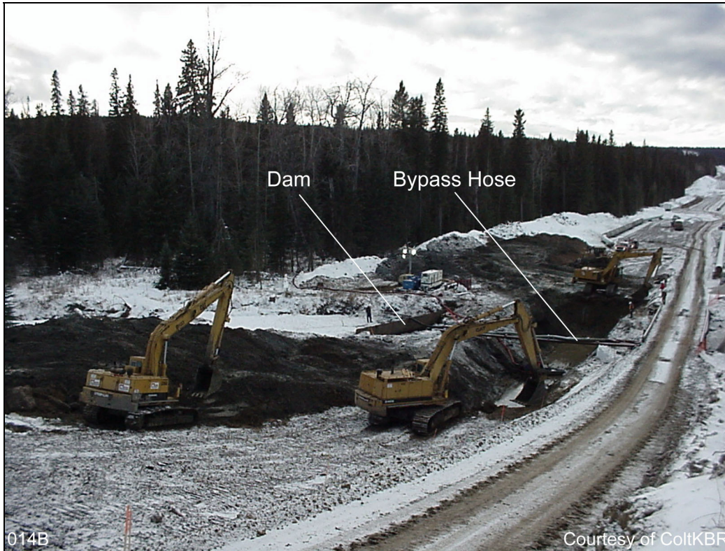
Figure 3-35: Example of Isolated Dam and Pump Crossing
