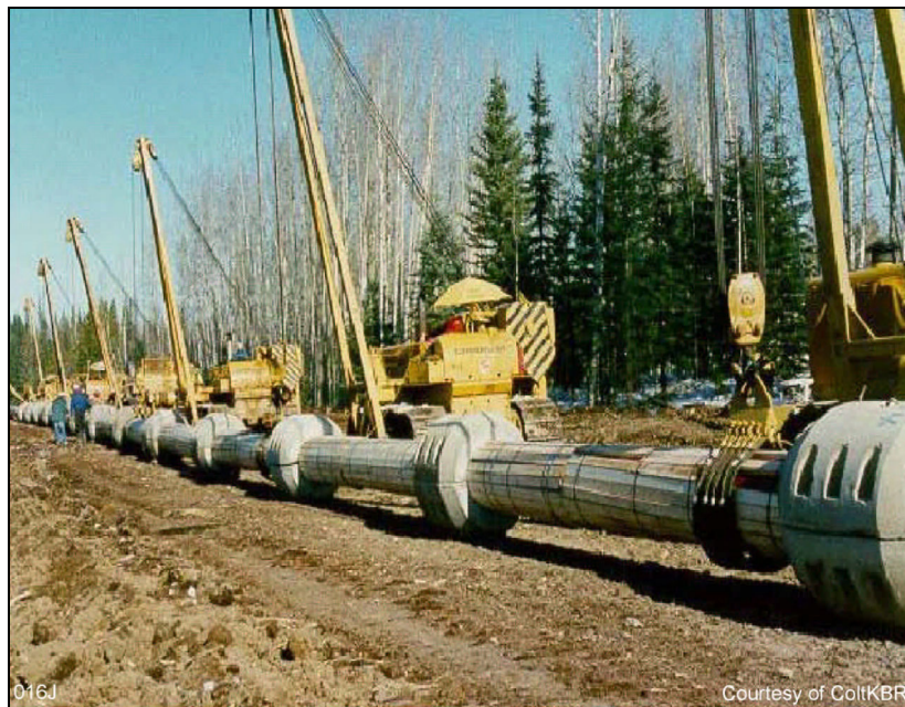
Figure 3-38: Example of Concrete Weights to Counter Buoyancy
