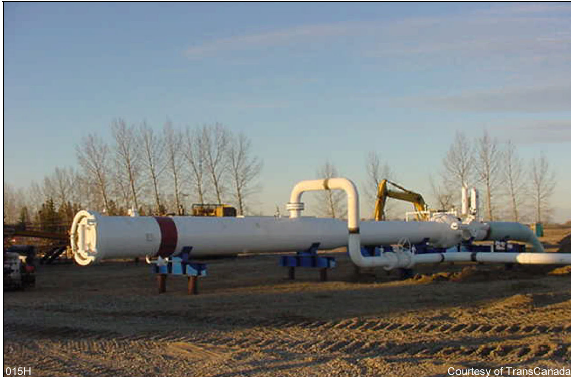
Figure 3-20: Example of a Pig Launcher or Receiver
