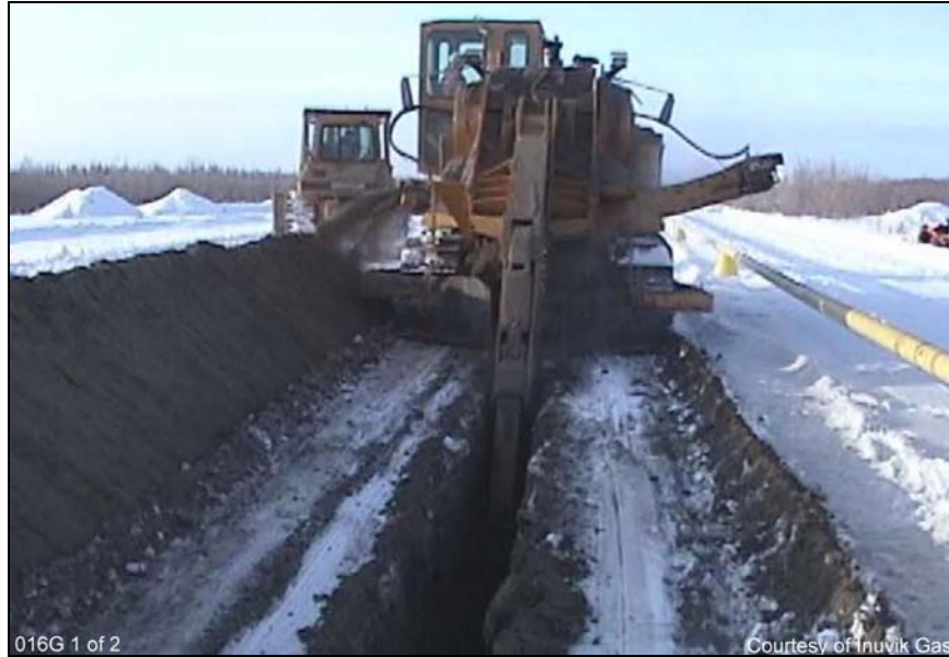
Figure 3-34: Example of a Chain Ditcher
