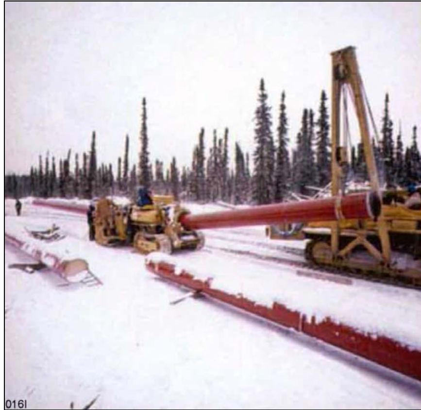
Figure 3-32: Example of a Pipe Bending Machine on Pipeline Right-of-Way
