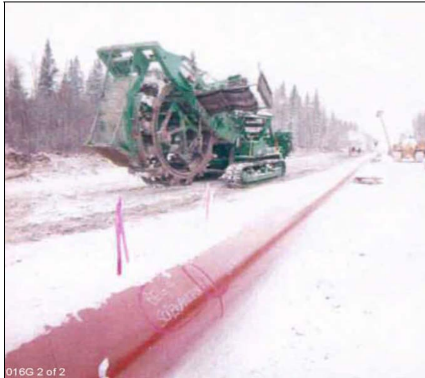
Figure 3-35: Example of a Bucketwheel Ditcher
