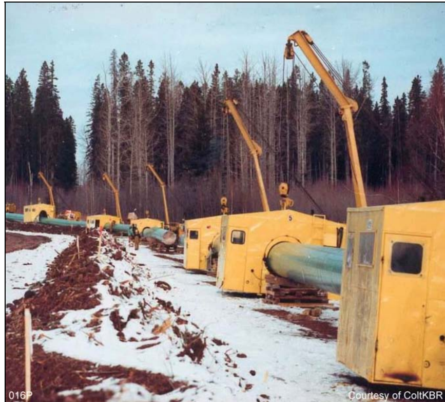
Figure 3-33: Example of Welding Shelters on Pipeline Right-of-Way
