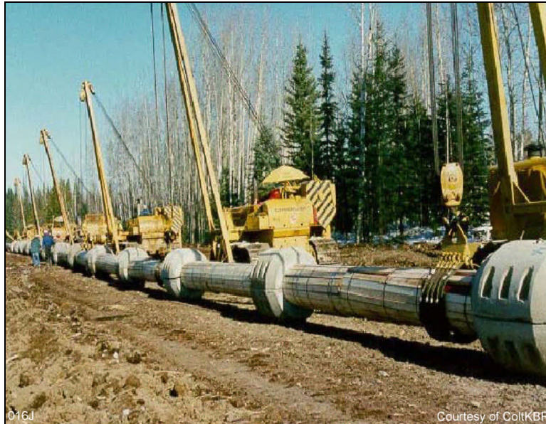
Figure 3-44: Examples of Concrete Weights to Counter Buoyancy
