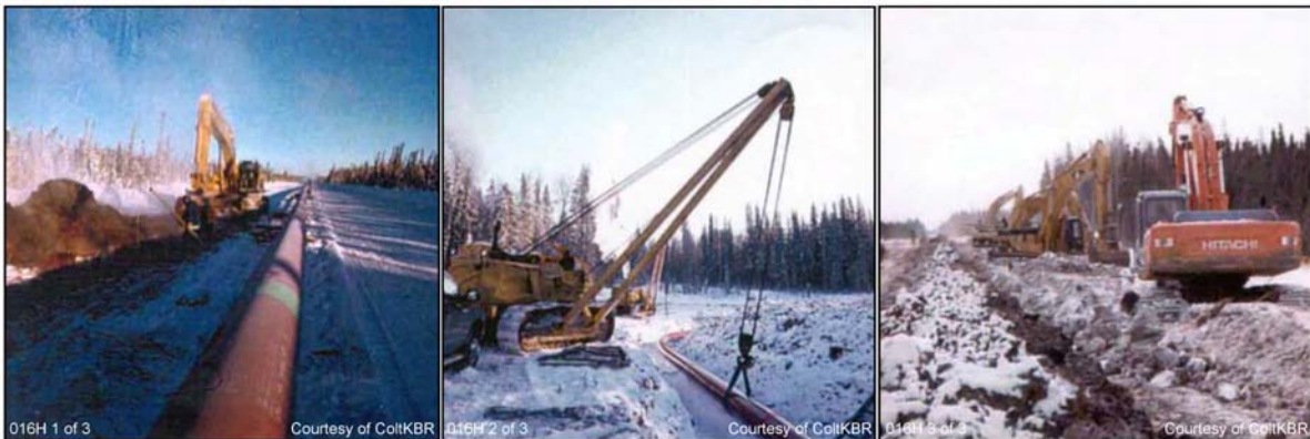
Figure 3-36: Examples of Trenching, Lowering in Pipe and Backfilling Cleanup
