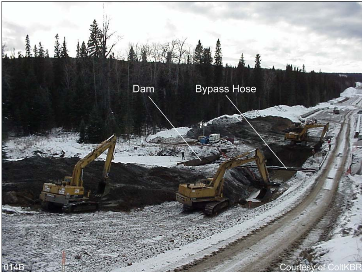
Figure 3-39: Example of Isolated Dam and Pump Crossing
