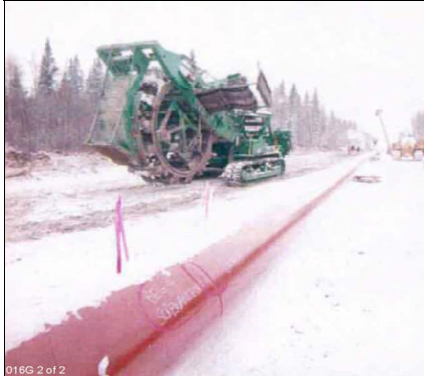
Figure 3-35: Example of a Bucketwheel Ditcher
