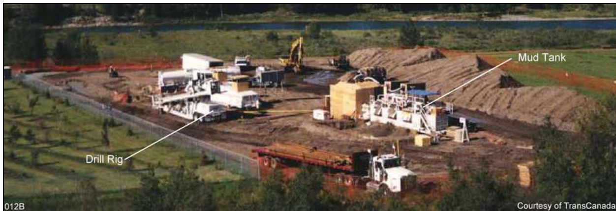
Figure 3-42: Horizontal Directional Drill Photograph – Entry Side
