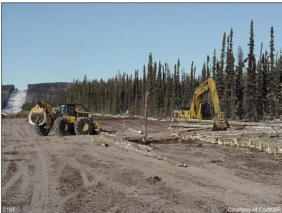
Figure 3-31: Example of Laying Log Corduroy on Travel Lane
