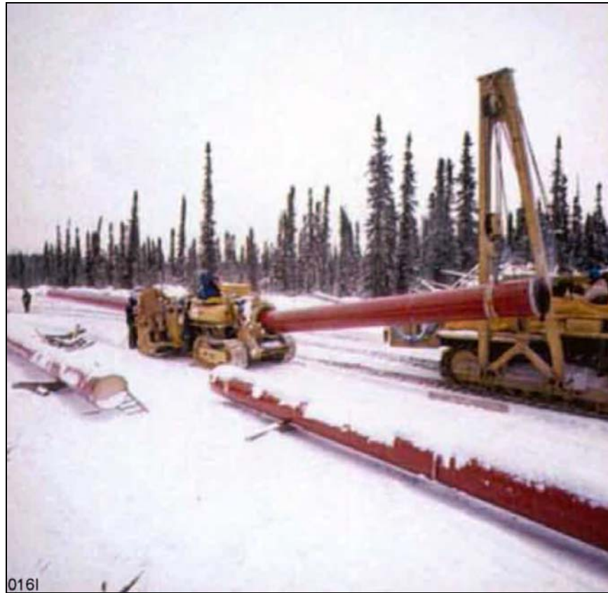
Figure 3-32: Example of a Pipe Bending Machine on Pipeline Right-of-Way
