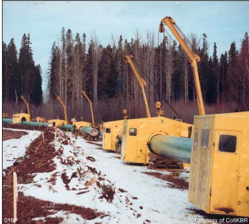
Figure 3-33: Example of Welding Shelters on Pipeline Right-of-Way
