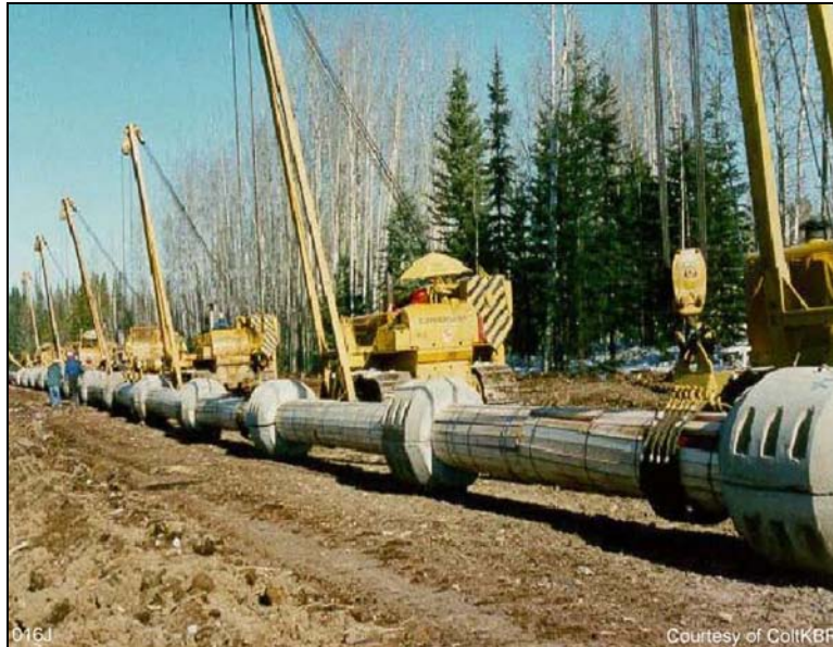
Figure 3-44: Examples of Concrete Weights to Counter Buoyancy
