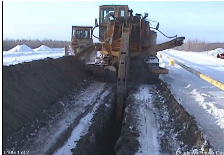
Figure 3-34: Example of a Chain Ditcher
