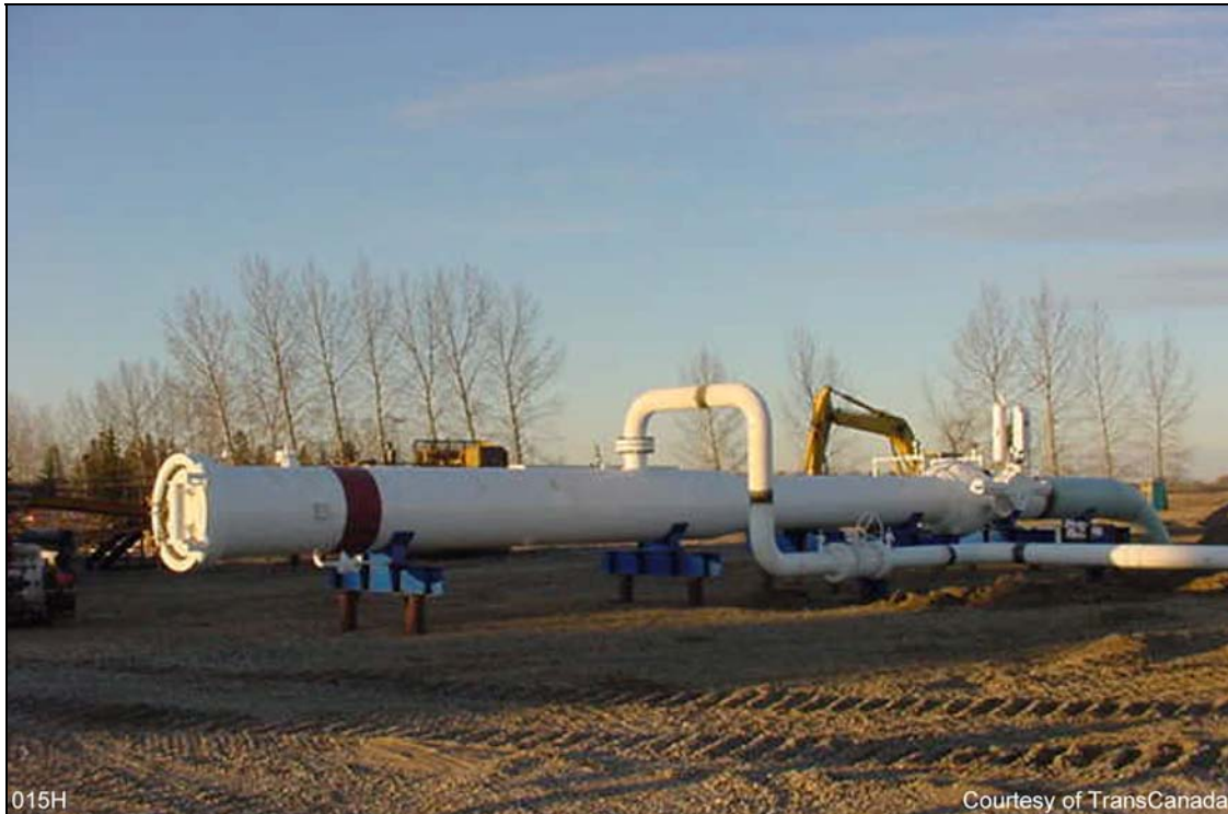
Figure 3-20: Example of a Pig Launcher or Receiver
