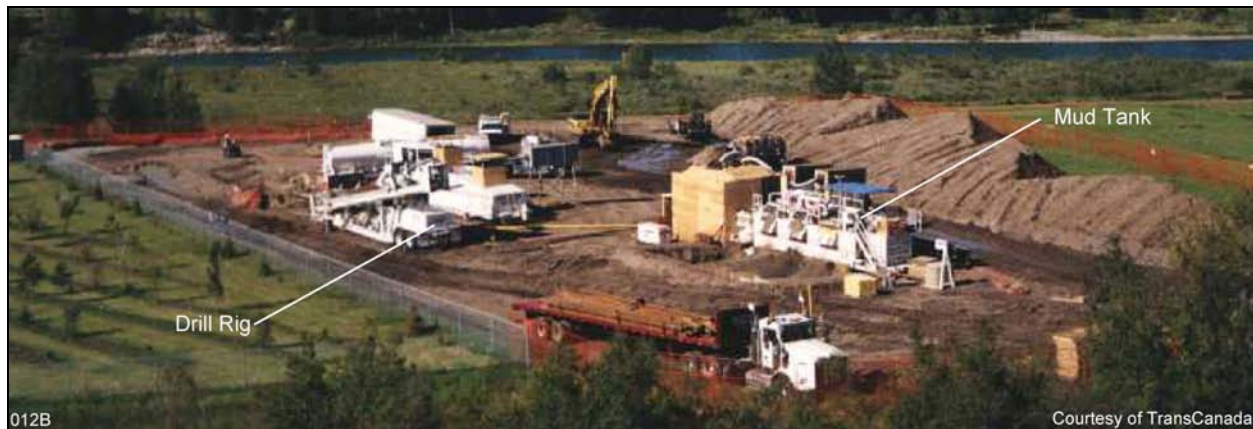
Figure 3-42: Horizontal Directional Drill Photograph – Entry Side
