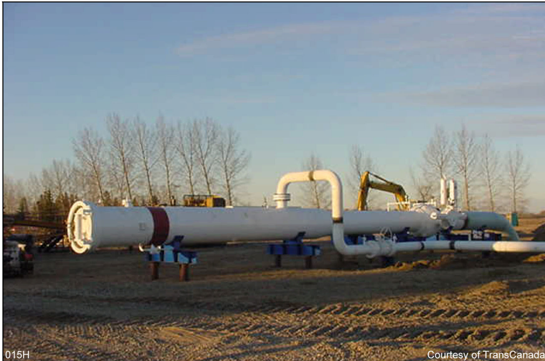
Figure 3-20: Example of a Pig Launcher or Receiver
